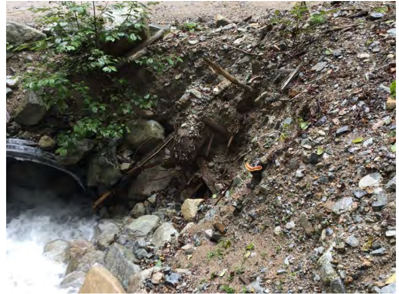
Right bank inlet armoring consists of material smaller than what the stream transports, plus organic material
