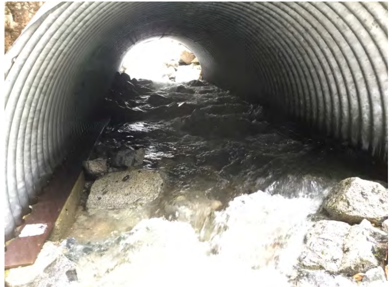
Looking through culvert from outlet
